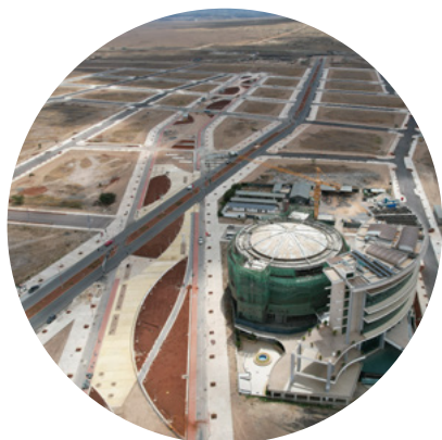
TECHNITAL, EPCF FOR INFRASTRUCTURE DEVELOPMENT OF KONZA TECHNO CITY, KENYA
