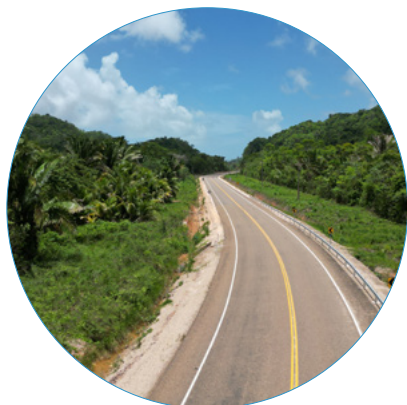
POLITECNICA, SIXTH ROAD COASTAL HIGHWAY UPGRADING PROJECT, BELIZE
