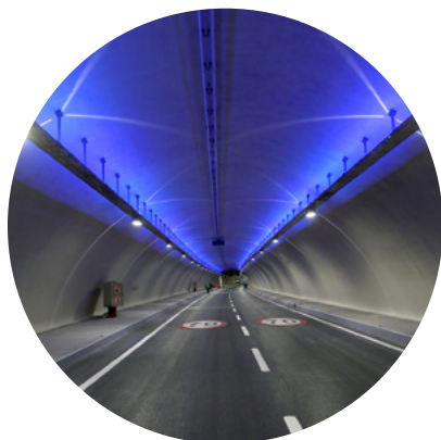
ITALFERR, EURASIA TUNNEL, TURKEY
