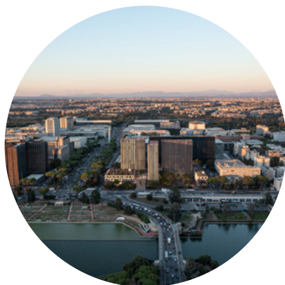
ARTELIA, ROME EUR TOWERS REDEVELOPMENT, ITALY
