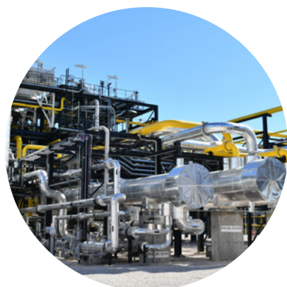
MAIRE, ZCINA TRAIN 4 LPG PROJECT, ALGERIA
