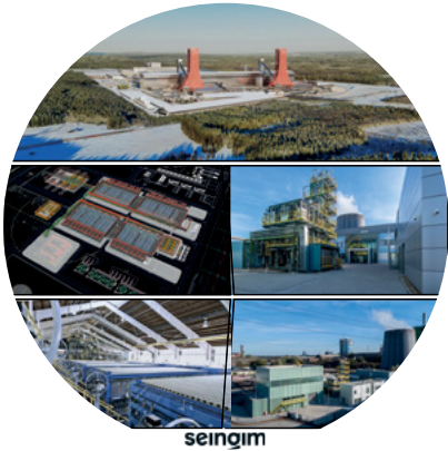
SEINGIM, HYDROGEN PRO- DUCTION PLANT, NORTH EUROPE
