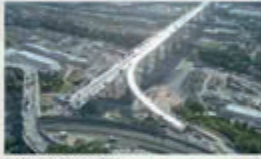
Genoa Saint George Bridge - Italy
